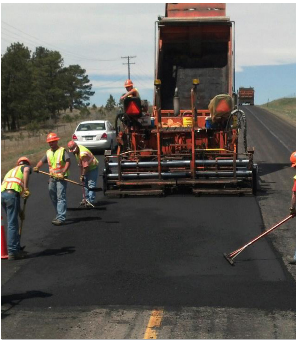
Construction on US 287 in Lamar.
