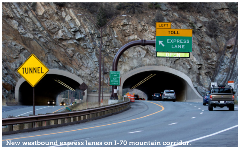
New westbound express lanes on I-70 mountain corridor.
