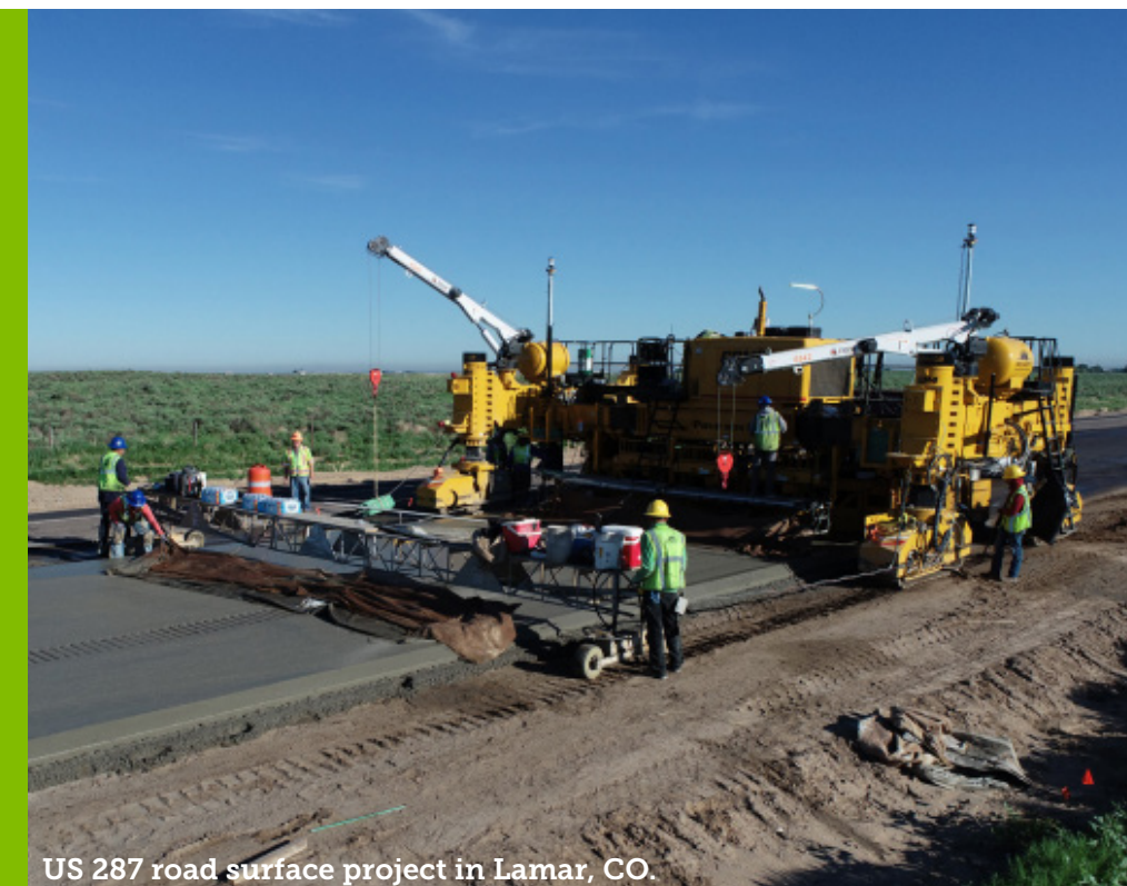
US 287 road surface project in Lamar, CO.
